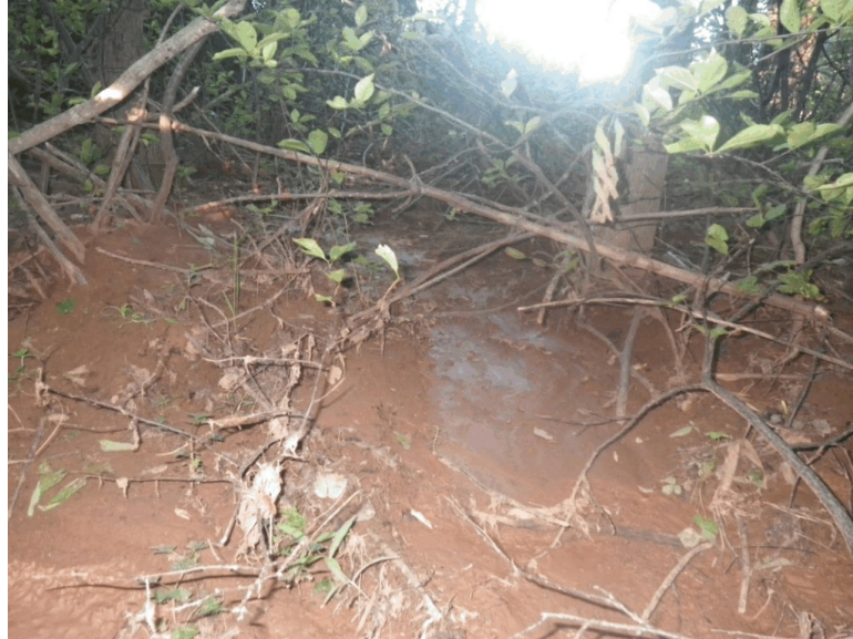
Figure 4. Sediment deposited in the flood plain of Campbellton Creek, upstream from the Coughlin Road. July 23, 2017
