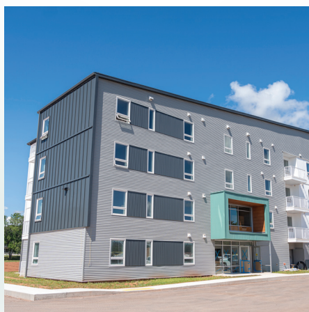
Summerside apartment construction
