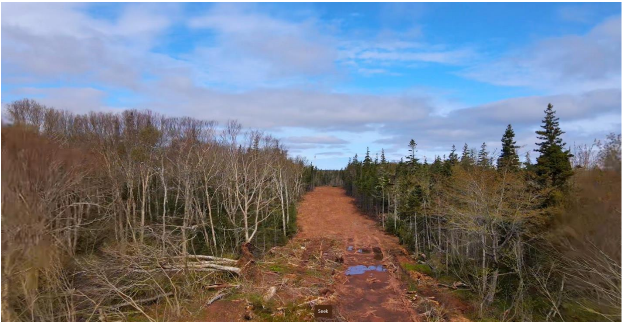
FURTHER DOWN THE ROAD IS A DUBIOUS WET SPOT.
